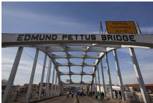
The historic Edmund Pettus Bridge in Selma, Alabama.
